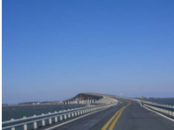
Figure 13. The Bridge between Middle and Lower Hooper Islands.
