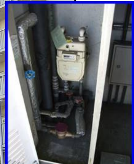
Internal of pipe-shaft
