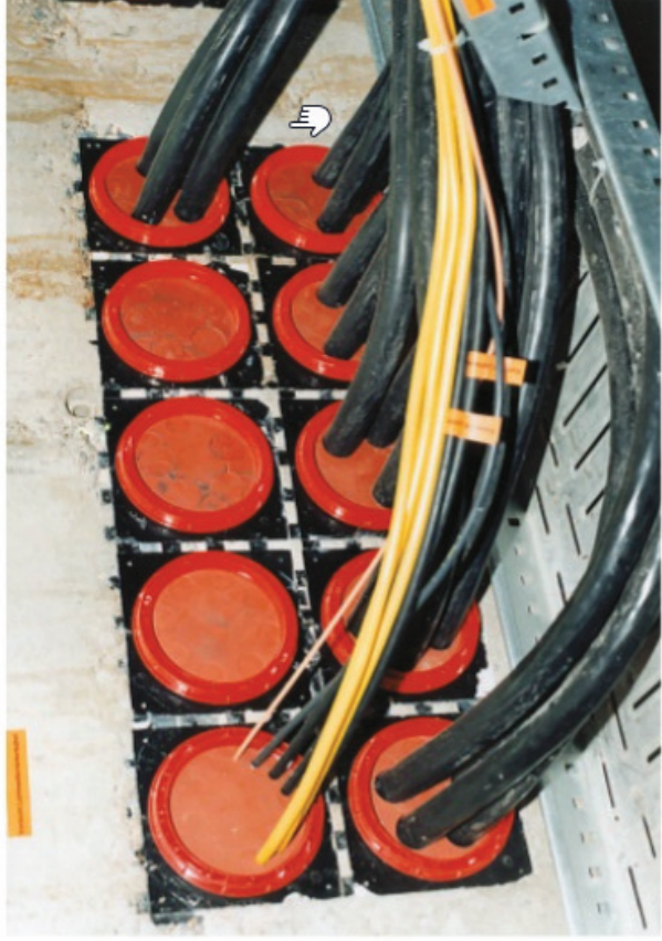
Cable penetration seal with modular seal
