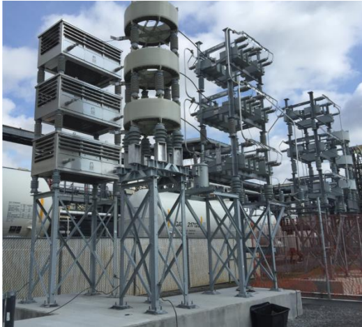
Stacked Reactor Arrangement
