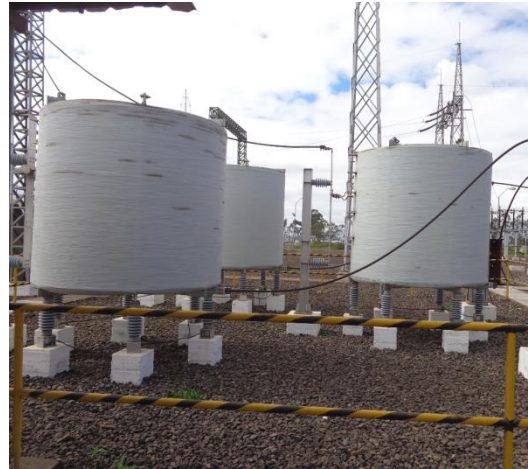
Unstacked Reactor Arrangement
