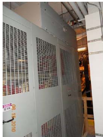
12.47kV snubber mounted horizontally above transformer
