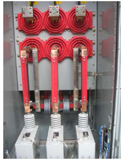
Fig. 19. Snubber for metal-enclosed 13.8-kV vacuum breaker.
