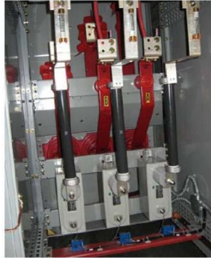
15kV snubber in MV switchgear (switchgear design)
