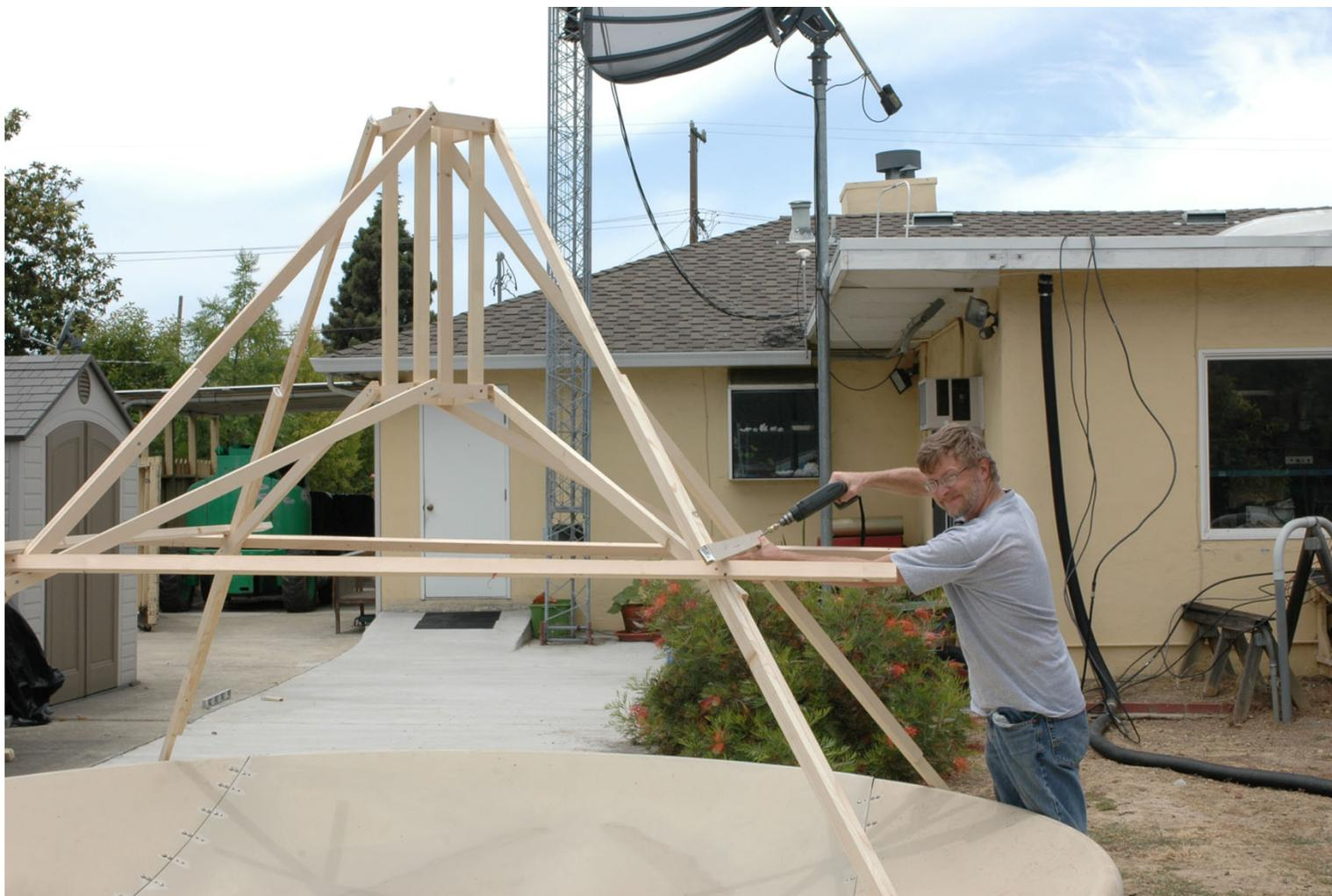
**Figure 20: Construction of the feed support structure**
