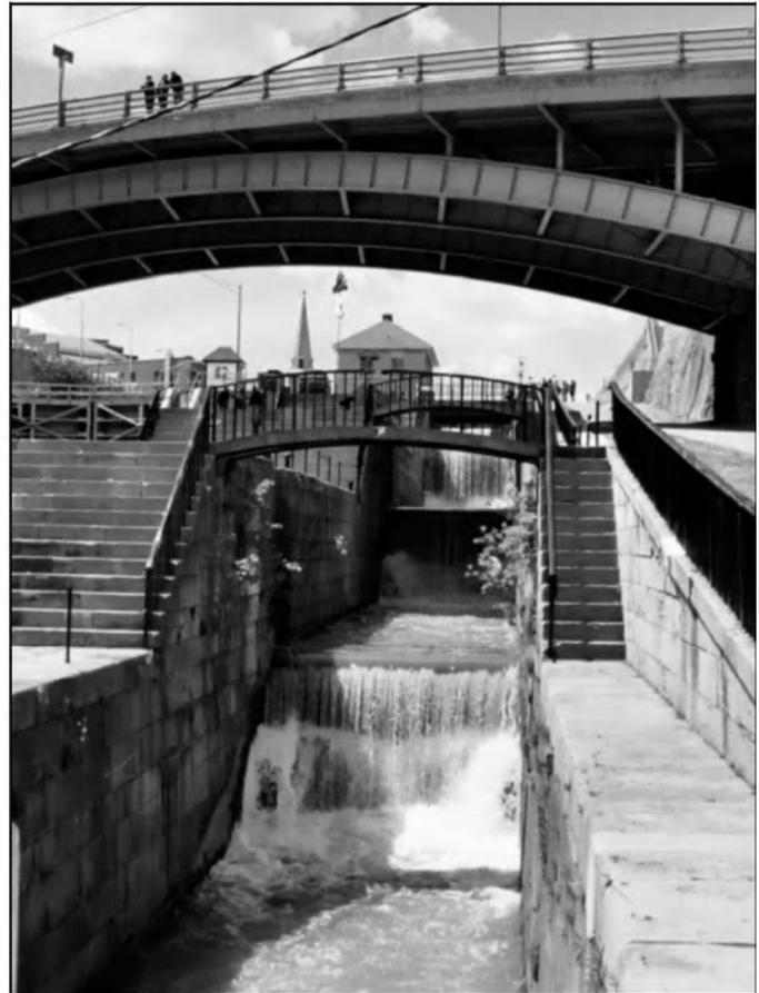
The original locks at Lockport have been replaced with one large lock, but the old ones remain as a spillway.
