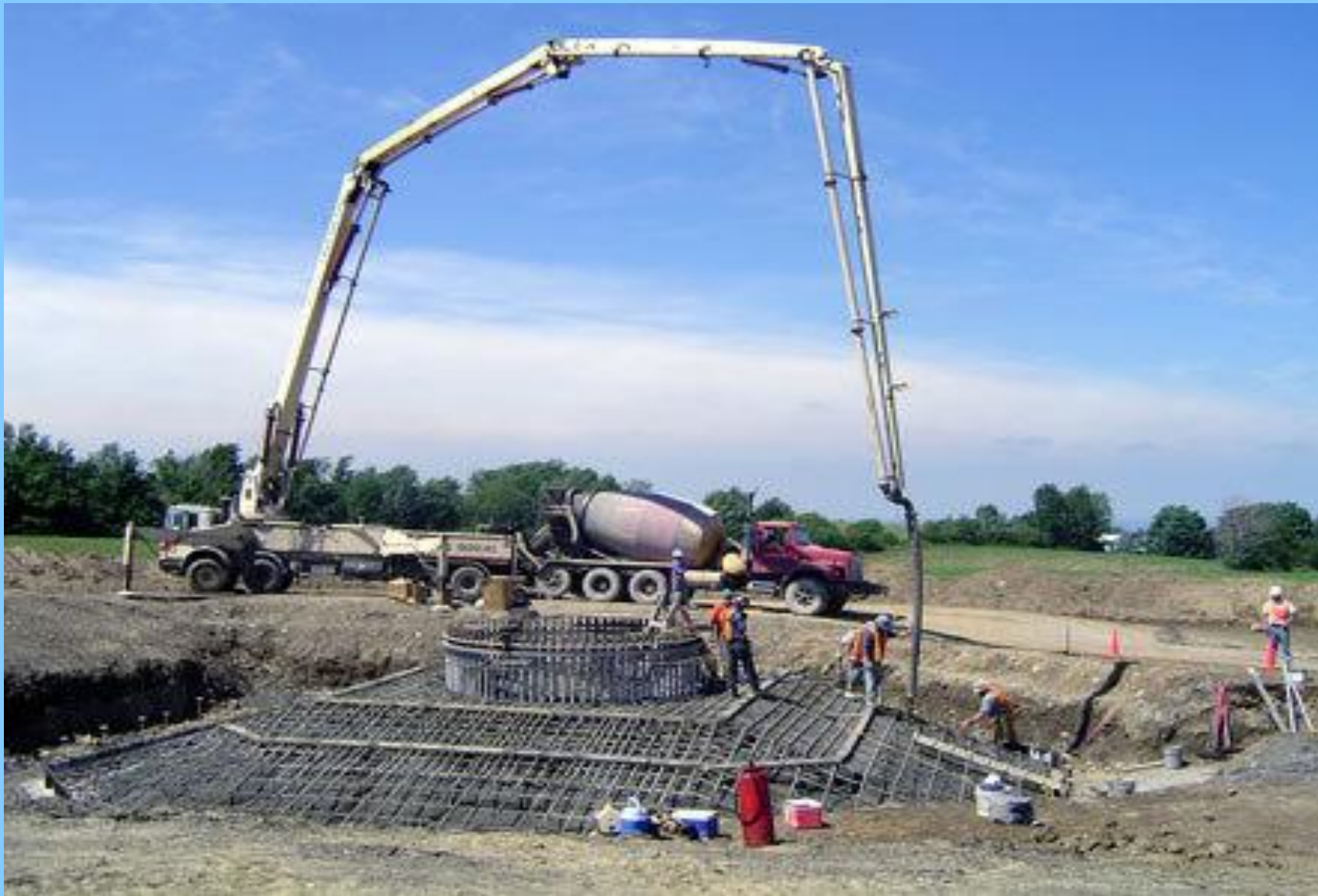
Pouring Concrete for the Base of a Windmill
