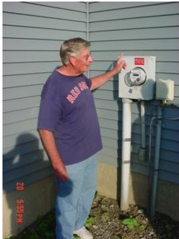
Roger explains details of the power distribution and smiles pointing to the power meter running in reverse, After all, it was a sunny day.
