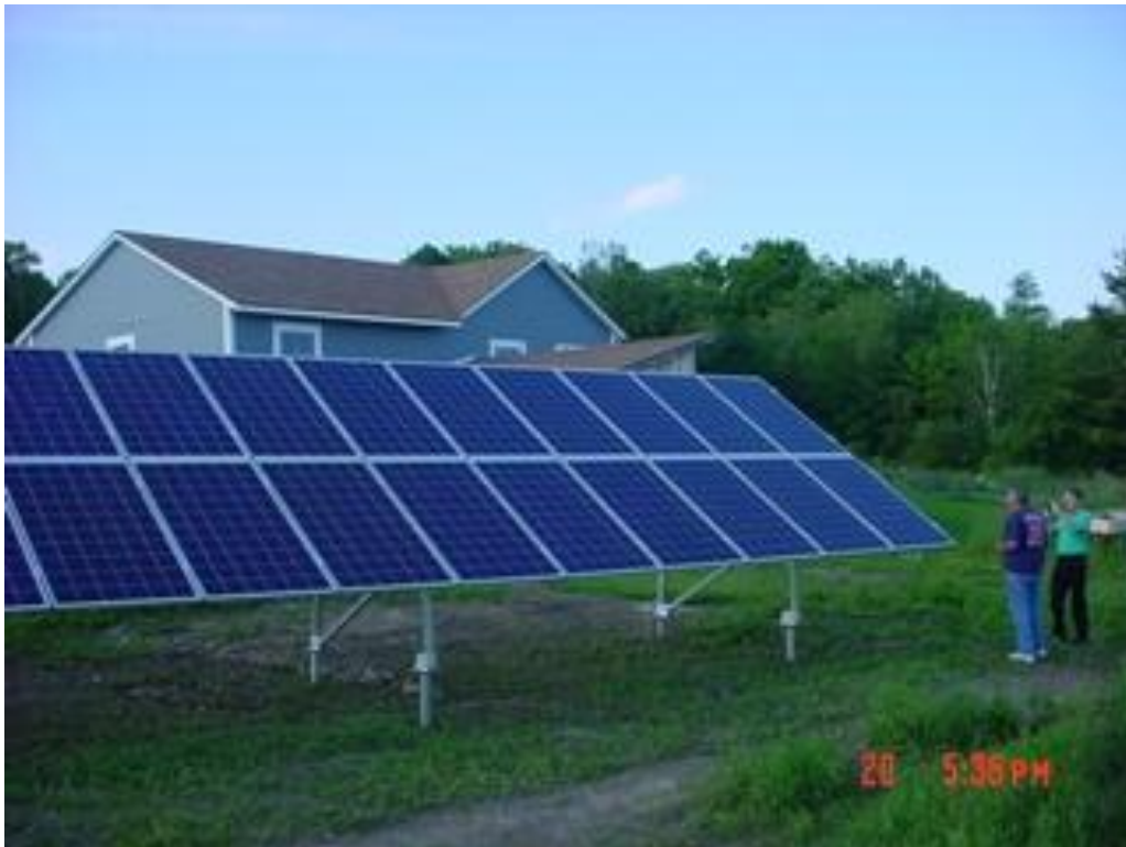
Roger Manzolini at his solar electric power system in operation, 40 panels, 8.6 KWatts – View 1
