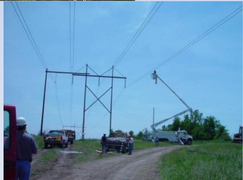
ENERGIZED 765KV SPACER RETRO-FIT
