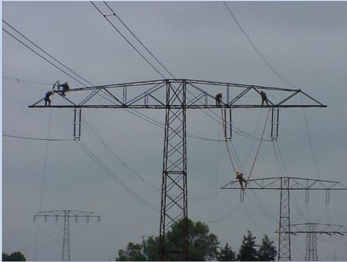
ENERGIZED 765KV SPACER RETRO-FIT
