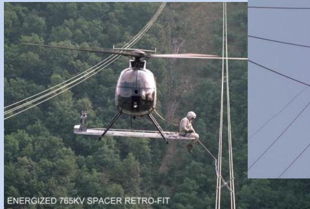
ENERGIZED 765KV SPACER RETRO-FIT
