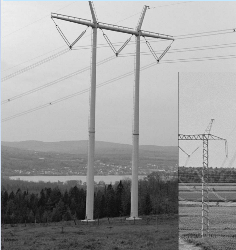
Figure 15.4-3 Hydro-Québec/TransÉnergie tubular self supporting tower.
