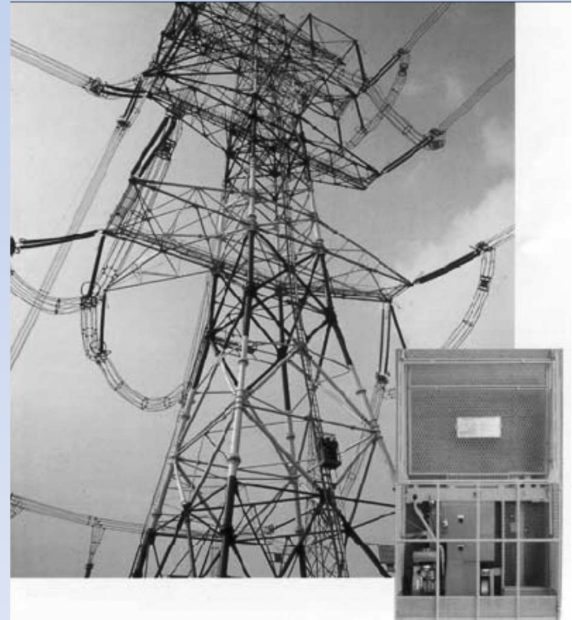
Figure 15.12-3 765-kV tower showing elevator and its rail.
