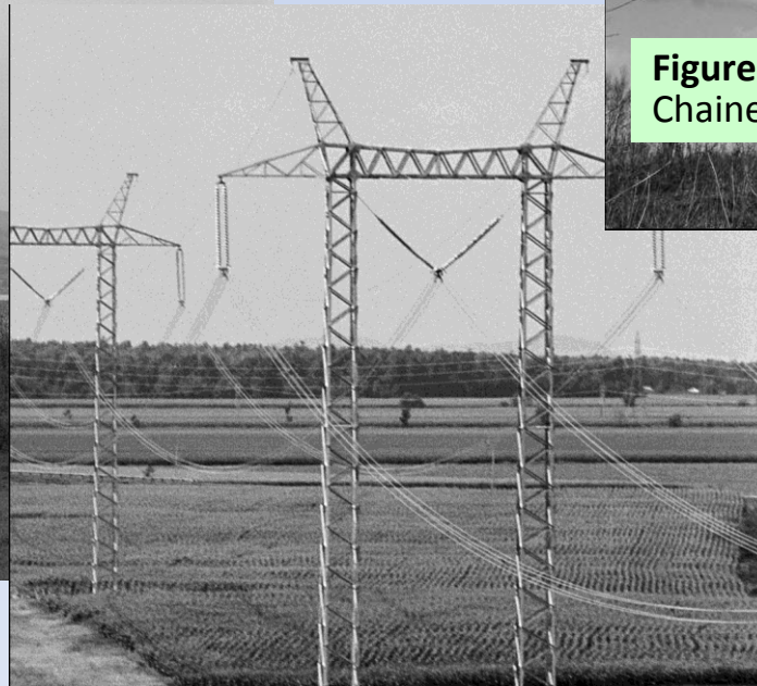
Figure 15.4-4 Hydro-Québec/TransÉnergie reinforced lattice steel tower.
