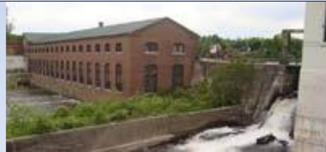
Mechanicville Power Station, Mechanicville, New York 1897
