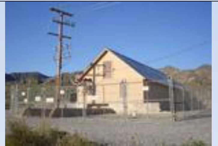
Redlands Mill Creek 1 powerhouse Redlands, CA 1893
