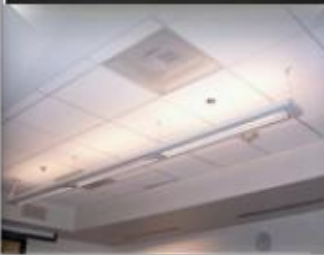
Southern Cal Edison Utility Services Office Irwindale, CA
