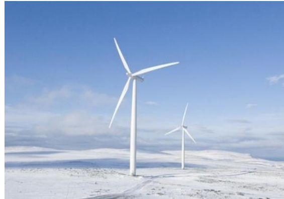
1.6 MW Wind Turbines
