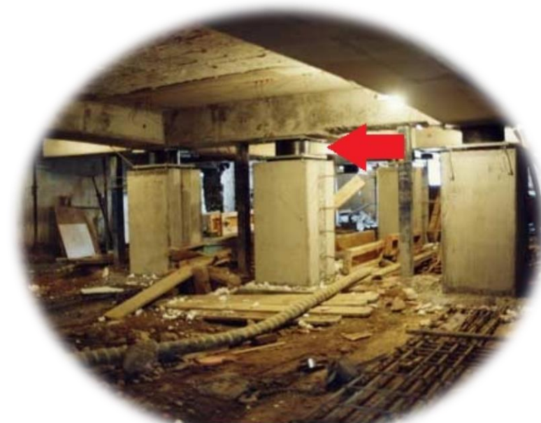
Old foundation with base isolator
