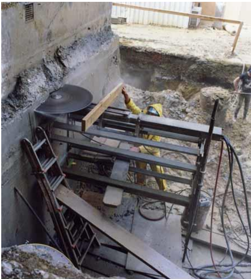
Cutting into the original foundation
