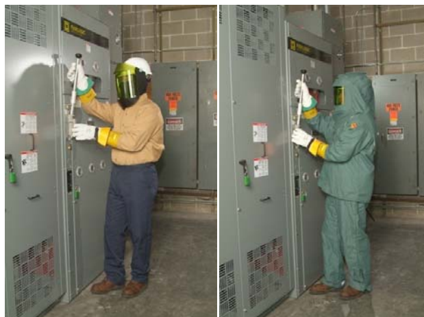
Fig. 1. PPE rated 8 cal/cm 2 (L) & 40 cal/cm 2 (R). Photos courtesy of Oberon.
