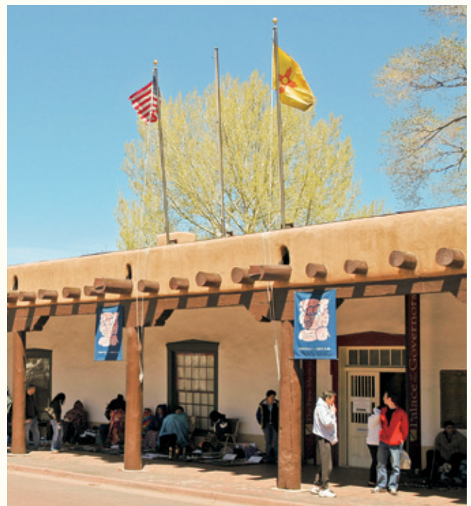
The Palace of the Governors, built in 1609, was previously the capitol building but is now the state history museum and a Registered National Historic Landmark.
