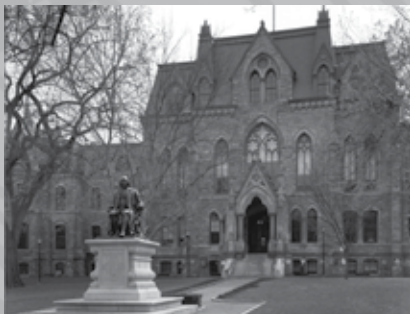
University of Pennsylvania Historic Stone Facade Repairs
