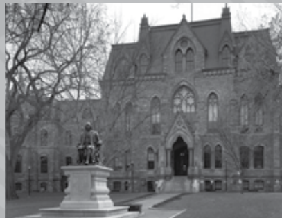
University of Pennsylvania Historic Stone Facade Repairs
