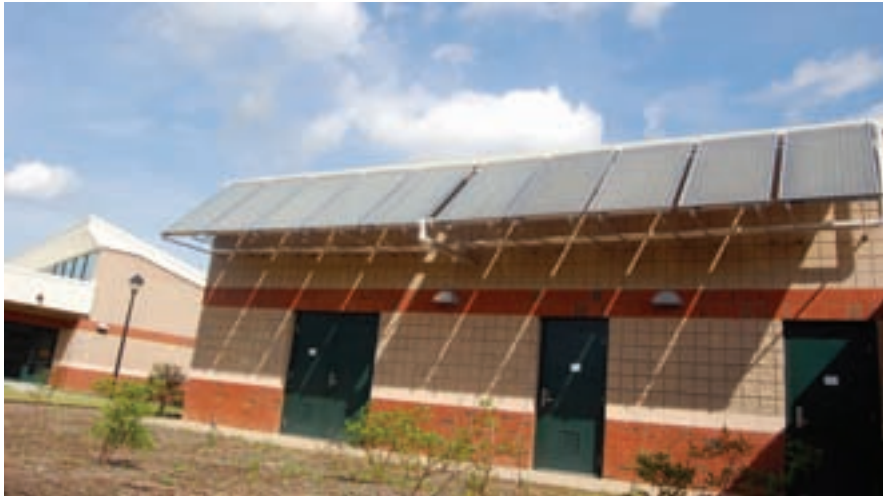
About 75% of Northern Guilford Middle School's hot water is provided by solar power from 10 compound parabolic collector panels. The school also gathers energy for a road sign and wetland aerators from three photovoltaic solar power systems.
