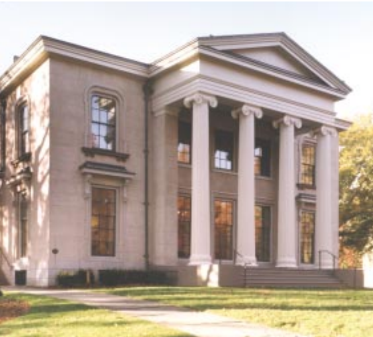
The east facade of the mansion shows the restored ceremonial stairs and double-height Ionic columns of the east portico. To the left, the south portico features fluted Doric columns and stone steps with an iron balustrade. Photo copyright © by Peter Mauss/Esto.
