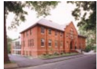
Main entrance facade with restored Gothic portal and sloped access sidewalk, and West facade with new connector addition. Photo by John Horner.
