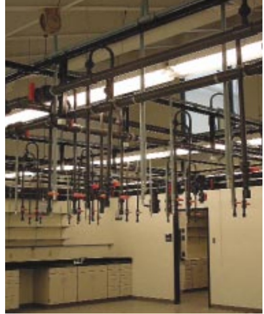
Laboratory with overhead seawater system. Photo by Van Dam & Renner Architects.
