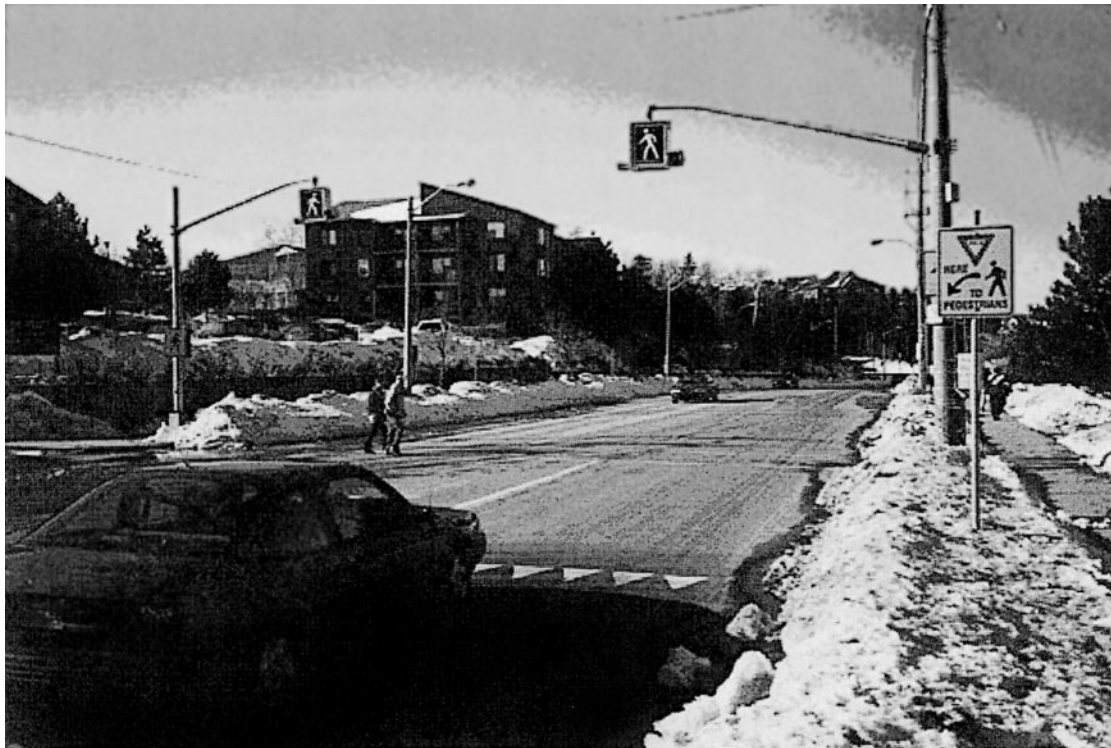
Figure 2. A picture showing a typical application of the advance yield markings and sign.
