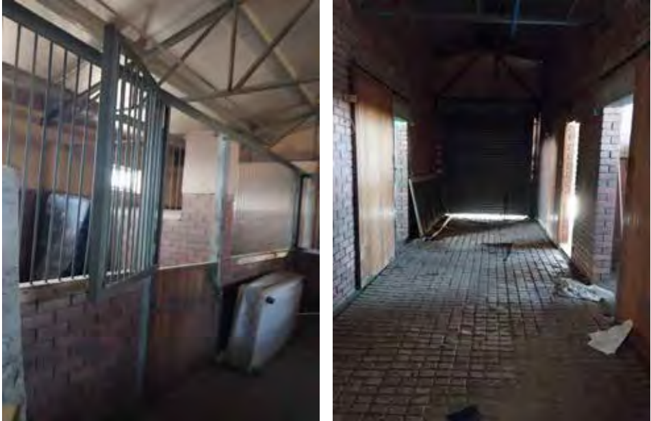
Figures 1 and 2: Building condition before renovation
