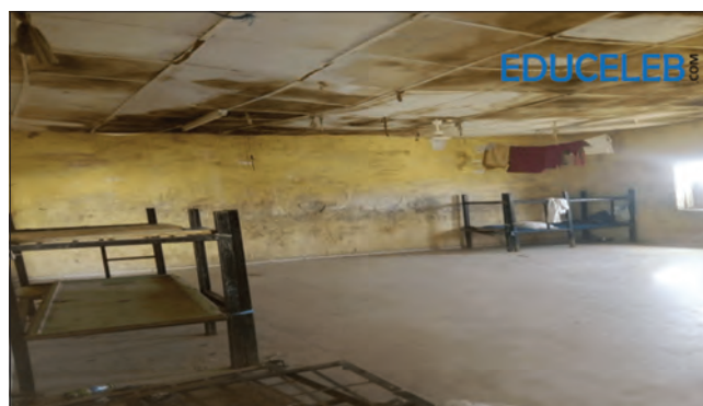
Figure 2: A typical hostel room in one of the schools. Source: Amoo (2019). Educeleb.com
