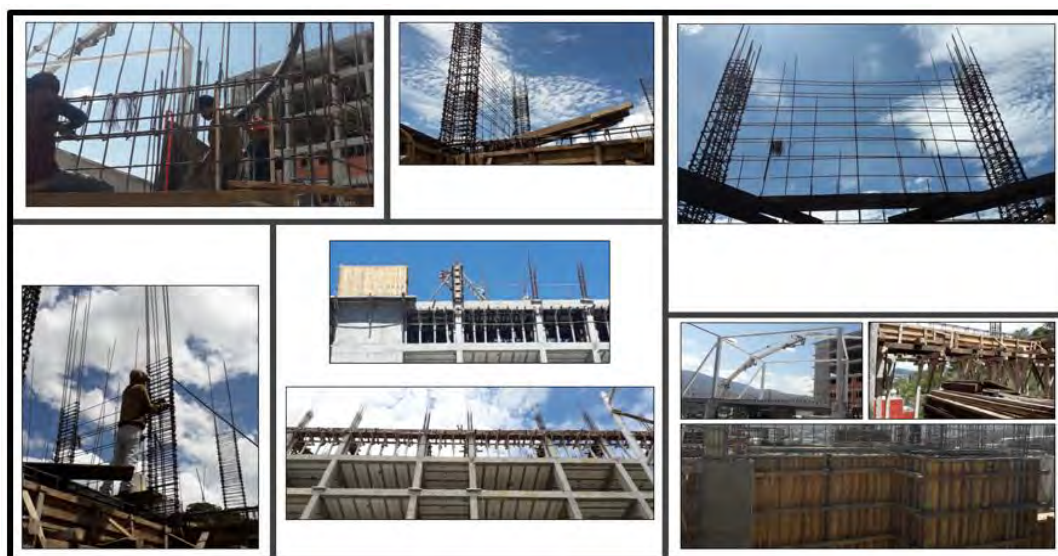
Figure 16. Photographs of buildings of civil engineering work
