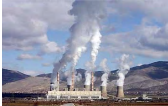
Figure 1. Photo of a real TPP (Kozani, Greece)
