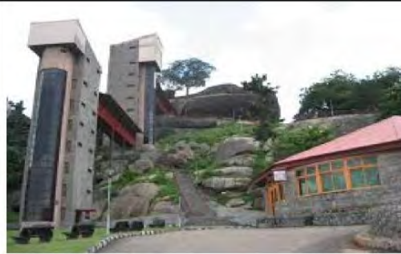
Figure 40. Uplifting of terrain of the Olumo rock environment
