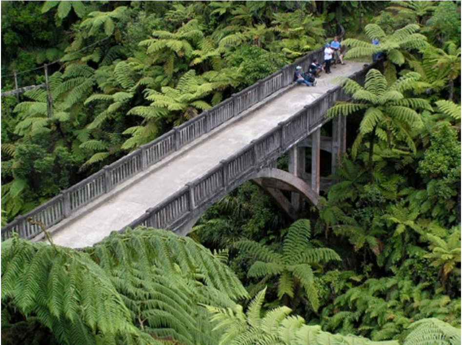
Figure 3. The Bridge to Nowhere. Photograph by J. Ebrey. Source: Creative Commons (Ebrey, 2005).
