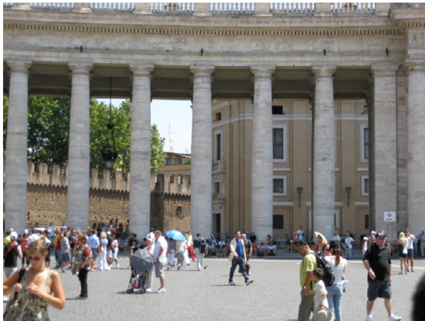
Standing at one of the foci of the elliptical colonnade, a visitor sees only the columns in the inner ring (the others are standing behind this first set along the line of sight). The city beyond is clearly visible. (Photograph taken by author.)
