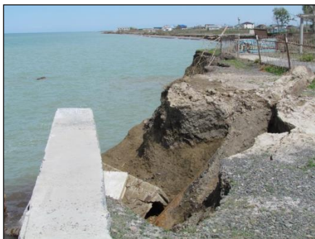
Figure 7. Destruction coast of Alakol lake and the negative impact of abrasion processes at village Kabanbay
