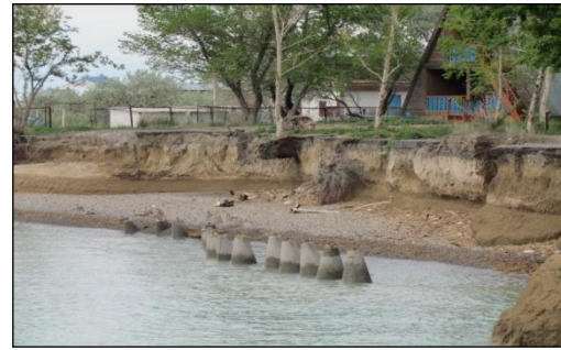
Figure 12. The breakwaters to protect the coastline of Alakol lake, village Kabanbay
