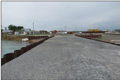
Figure 11. Pier to protect the coastline of Alakol lake, village Kabanbay
