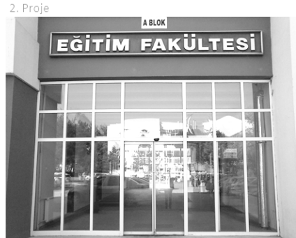
Figure 8. New entrance door of block A
