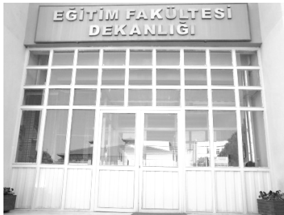
Figure 3. Entrance door of block A
