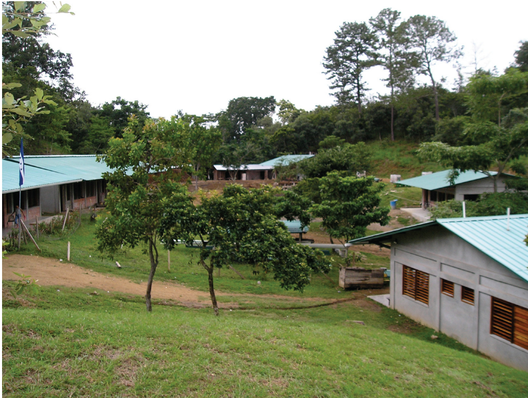
Figure 4: Bi-lingual elementary school campus under construction.
