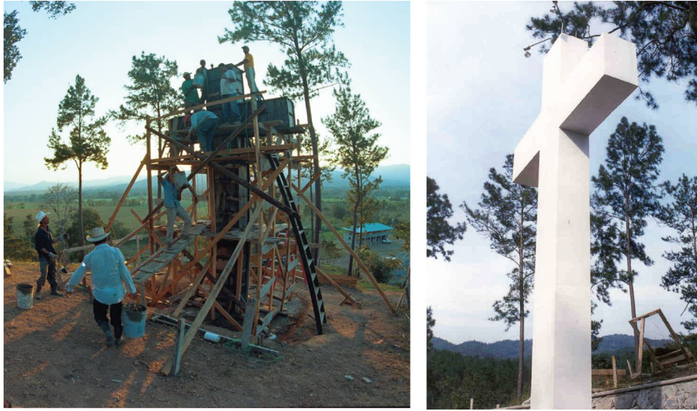
Figure 1: The concrete cross during construction and as it looks today.
