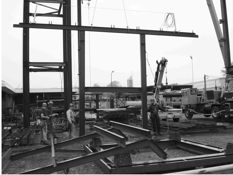
Figure 1. The four beams, assembled and being lifted.
