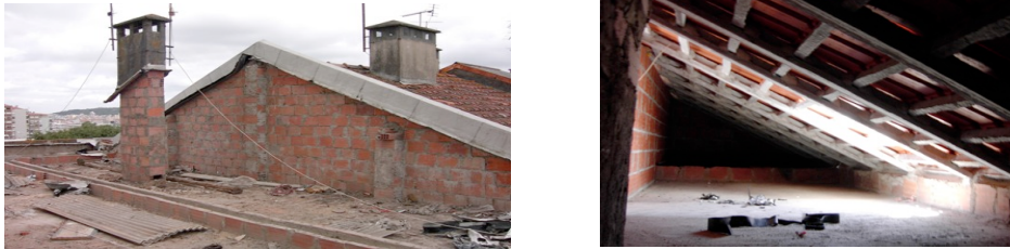
Figure 6. The interior and exterior view of the inclination of a gable roof.
