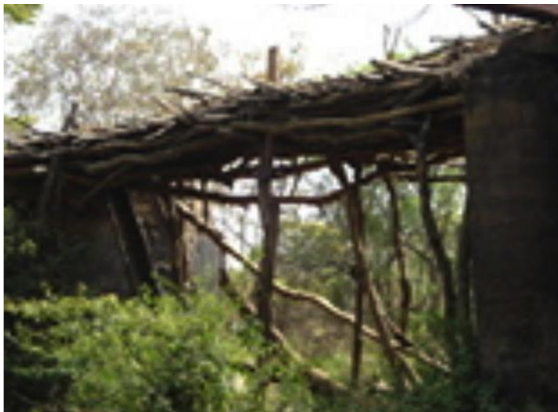
Figure 5. Sarah's picture of a wood bridge (June 24 th , 2012). Her narrative reads, "A bridge rarely found. This bridge is made of tree branches and mud. It is unbelievable that even the lorries use it. Local people made it after the falling of the permanent one. This shows how we can make use of available resources to do the impossible."
