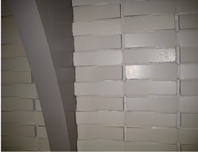
Image 5: Alta Vista Elementary School Addition, west end wall.
