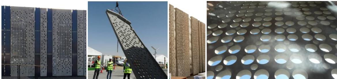
Figure 3. Left: Ultra-high performance fiber concrete (UHPFC) external layer as a solar shield, Center left: the precast UHPFC panel, Center right: the multilayered wall, Right: the porous UHPFC panel
