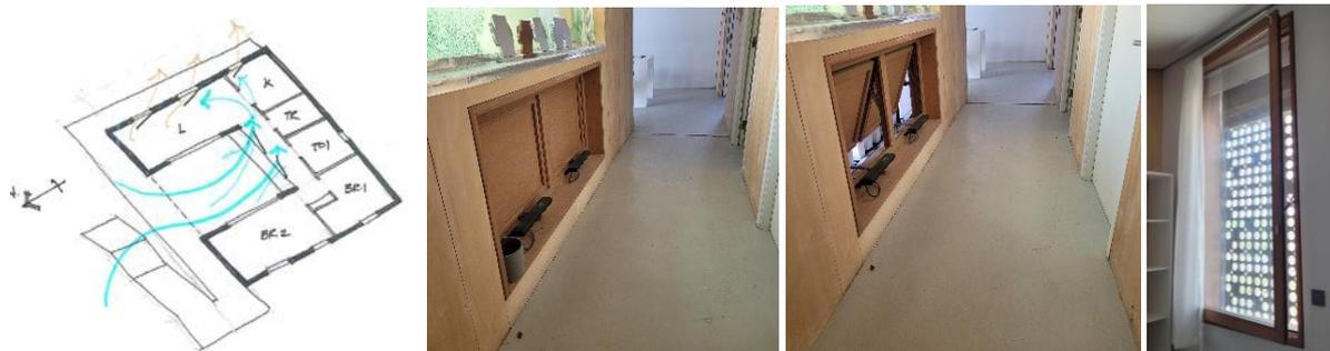
Figure 7. Left: plan view of Baitykool Living Lab with night ventilation strategy, Right: Image of Patio Ventilator with closed, open position & window in open position.
