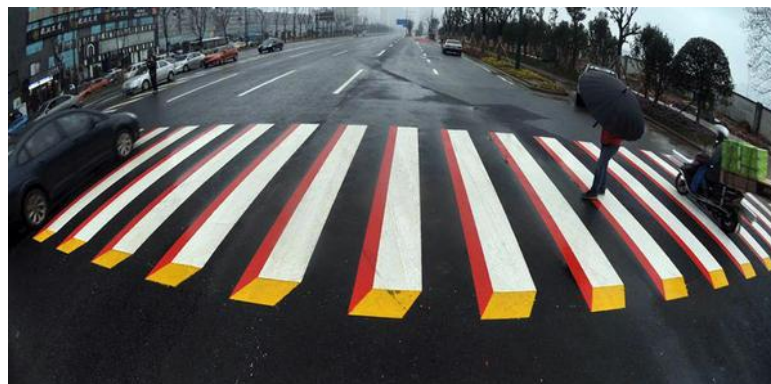
Figure 3. 3D Crosswalk in Delhi, India
