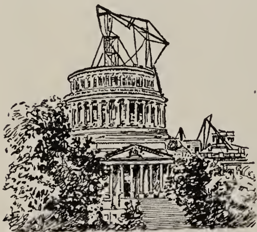
Building the present Capitol
