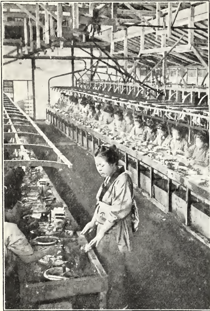
FIG. 151. Boiling cocoons and reeling silk in a great modern silk factory in Japan. These girls work long hours every day for a few cents. Much of the labor must be done by hand.
