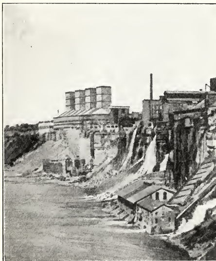
FIG. 194. Using the power of Niagara. The banks of the river below the Falls are lined with factories where a part of the tremendous power of Niagara is used. Some of the water may be seen returning to the river after turning wheels in the factories.
