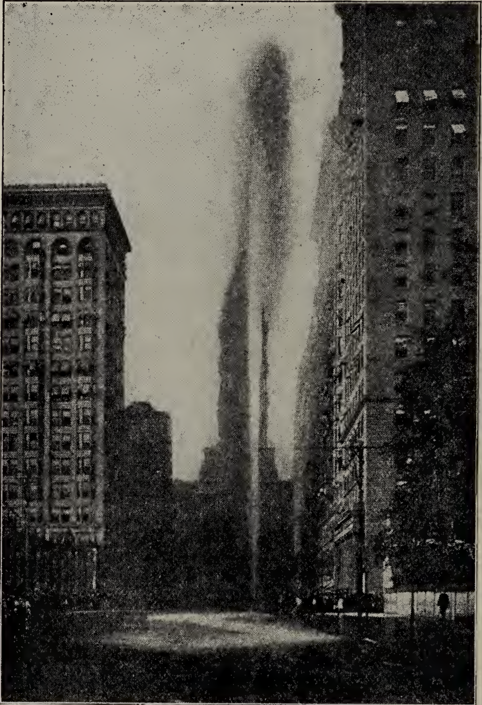
FIG. 248.—Philadelphia high-pressure fire service. Vertical stream made in underwriters' test.
