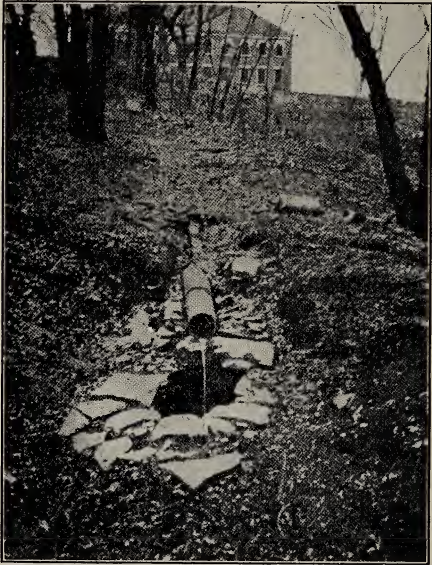
FIG. 264.—Pollution of ground water: sewage discharging into sink-holes.
