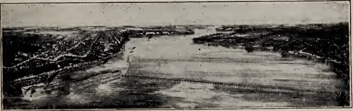
FIG. 296.—General view of the Mississippi River, the locks, the power house and the dam at Keokuk. The power plant is capable of producing 300,000 horse-power. It cost $25,000,000.
