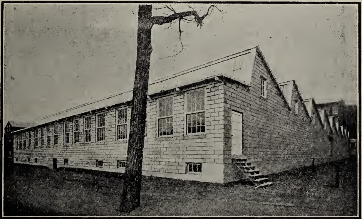
FIG. 35.—Weave shed at a cotton mill, showing the saw-tooth roof. We are looking at the northwest corner of the building; the roof windows face the north.
