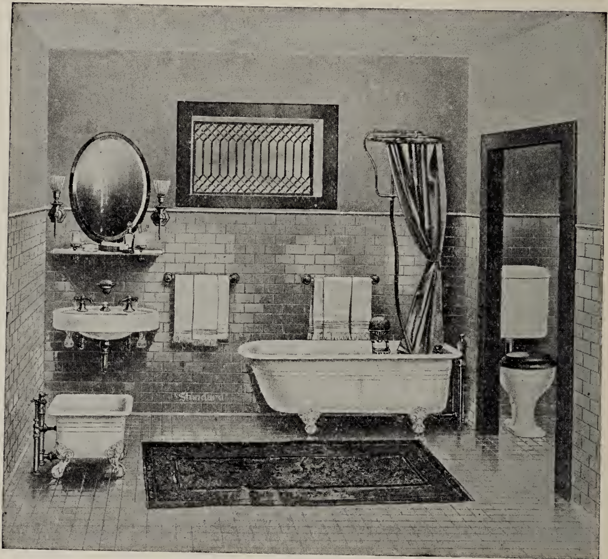
FIG. 261.—A modern sanitary bathroom.
