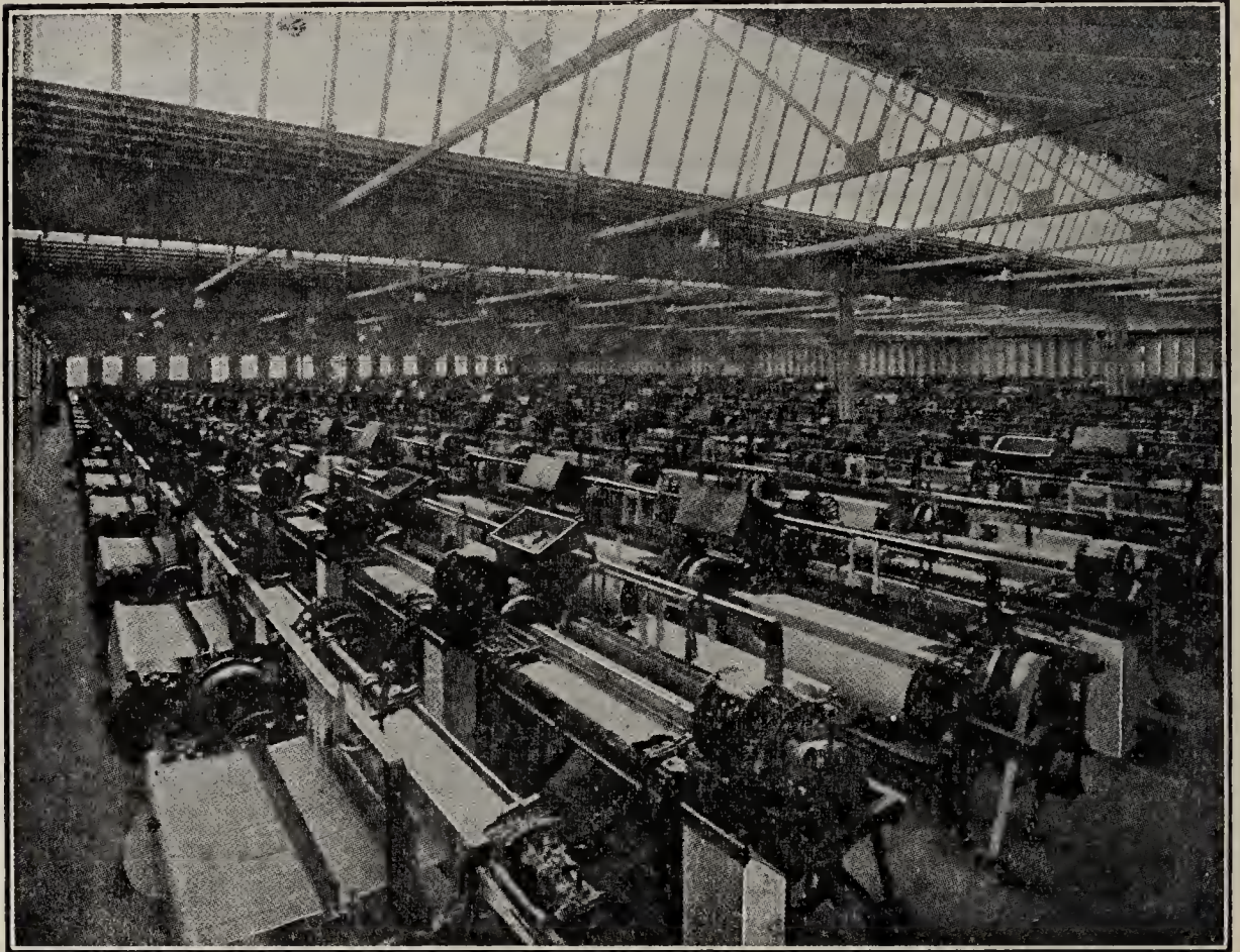
FIG. 36.—Interior view of the weave shed. The camera stood in the southwest corner of the room. Note the evenness of the lighting throughout the room. This room is 253 ft. by 140 ft. and contains 648 looms.
