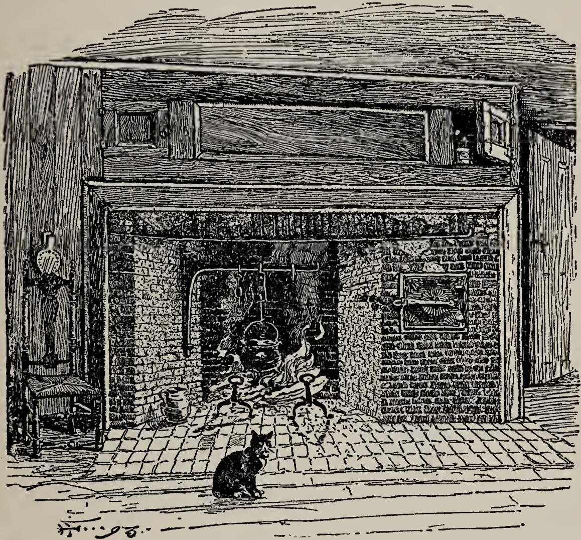
FIG. 59.—An old-fashioned fireplace and oven. (From Stories of Useful Inventions . By permission of The Century Company.)
