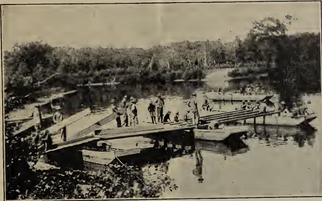
Pontoon bridges are built in quick time at Camp Devens, Mass.
