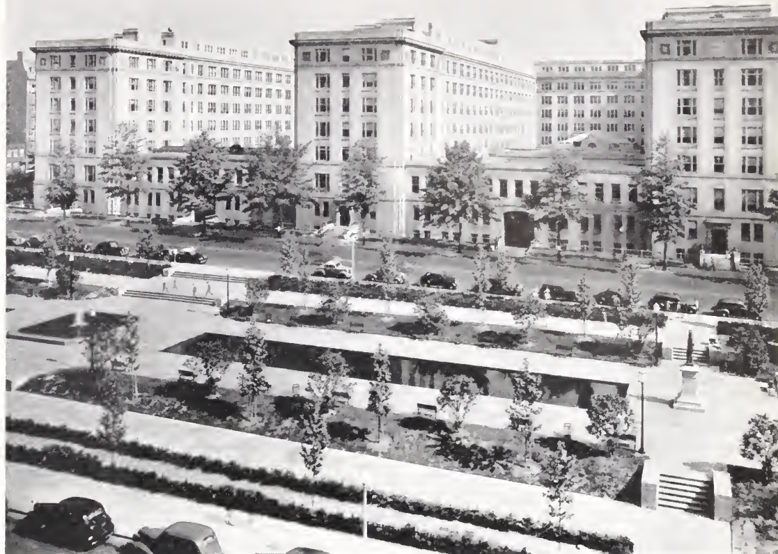
North Interior Building.
