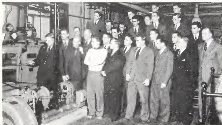
AIR CONDITIONING means more than mere comfort when applied to a submarine. That is why the University of New Hampshire is teaching it to these civilian employees of the Portsmouth Navy Yard.
