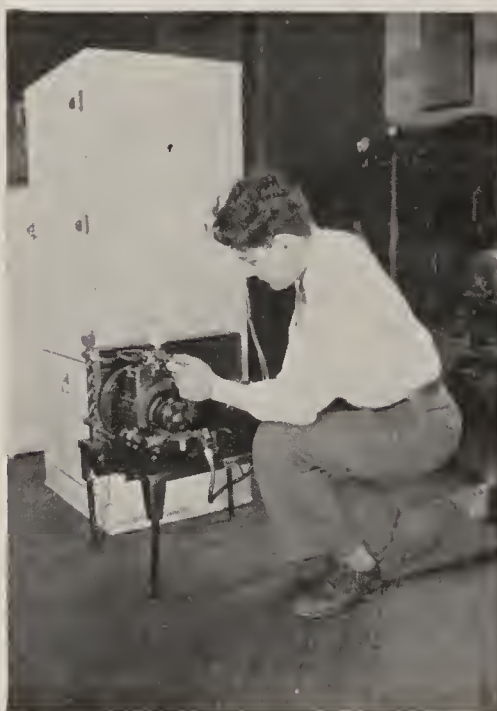
Adjusting a refrigeration unit in appliance servicing course, Allegheny Vocational School, Pittsburgh, Pa.
