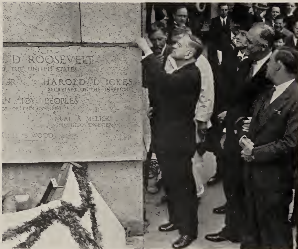
President Roosevelt and Secretary Harold L. Ickes, of the United States Department of the Interior, officiating at the cornerstone laying.
