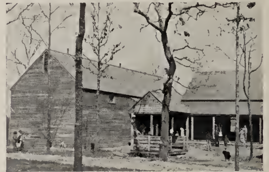
Temporary school building used by Cumberland homestead children. The building has been reconditioned by pupils and parents.
