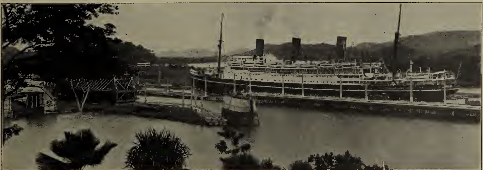
Courtesy of the Panama Canal
