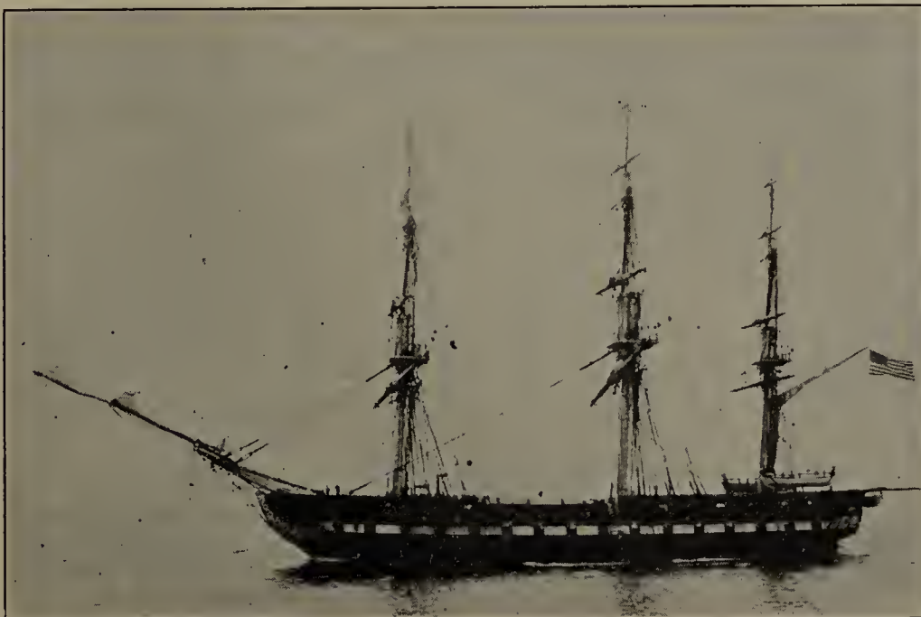
Courtesy Bureau of Construction and Repair, Navy Department
