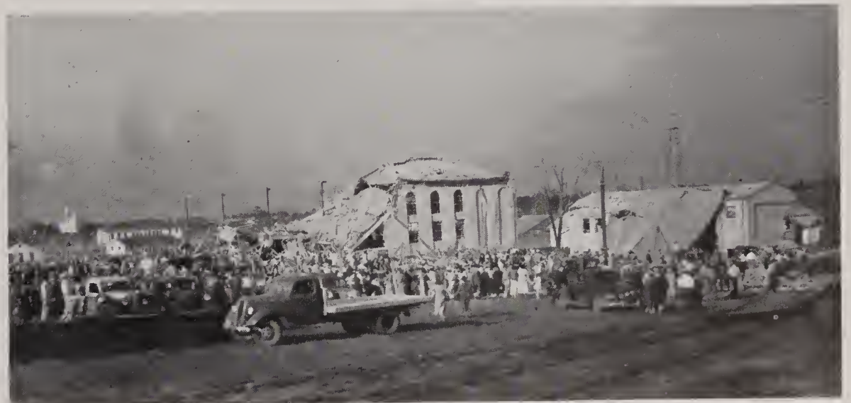
Ruins of the same building pictured below, after a tragic explosion occurred.
