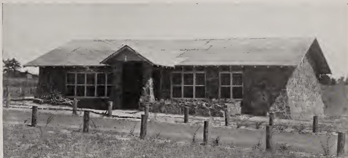
Better facilities such as this school building erected by five enrollees working during their spare time at Company 3782, CCC, Heber Springs, Ark., make possible better educational programs.
