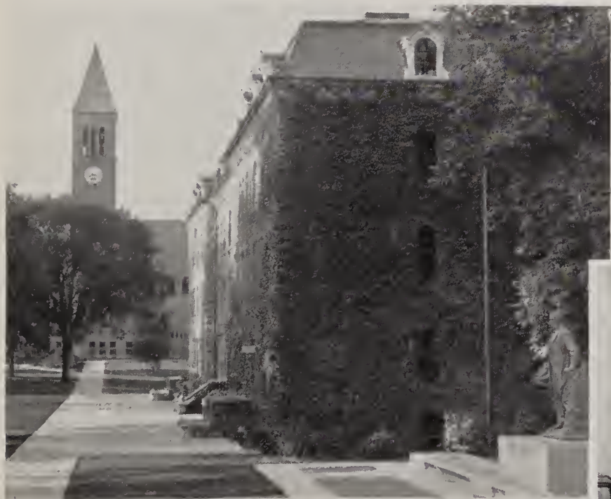
One building is usually designated as the administration building.
