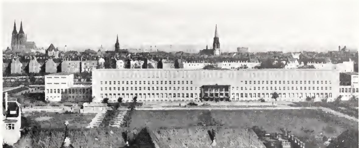
The new building of the University of Cologne.
