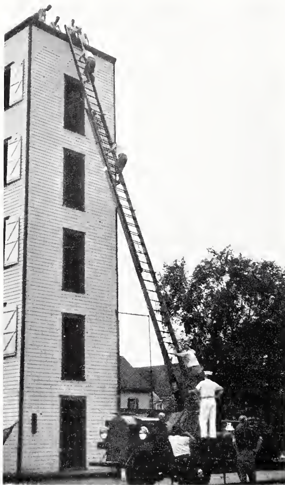
Firemen in Connecticut training class learning how to handle ladders on a drill tower built especially for training purposes.
