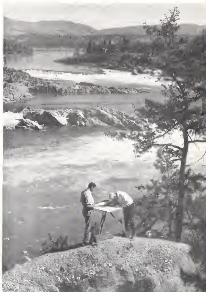
Surveyors plan the reservoir above Grand Coulee Dam which will supply water for irrigating 1,200,000 desert acres. Engineers and builders work night and day to complete the dam, the world's most massive masonry structure.
