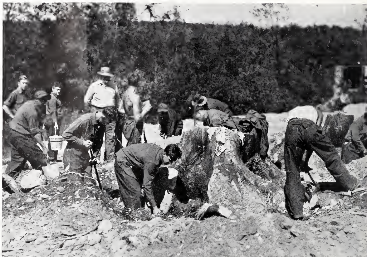
Clearing new ground.
