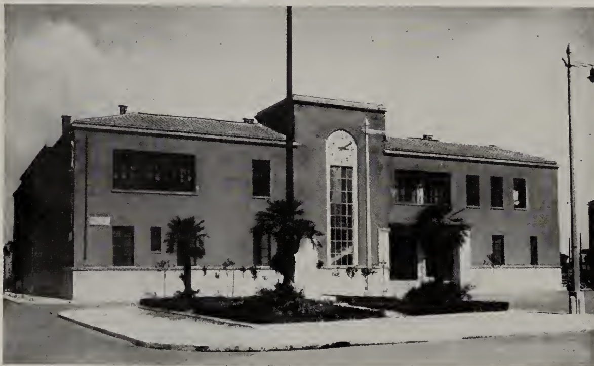
A communal school building at Littoria.
