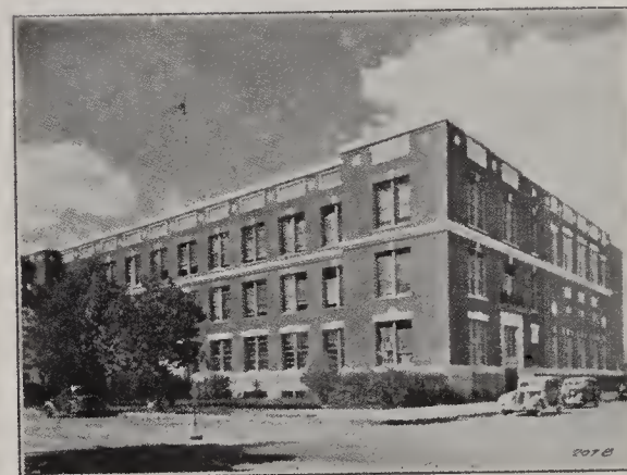
BUILDING (CLASS A) PUBLIC SCHOOL 207 BOROUGH OF BROOKLYN OCCUPIED JAN 11, 1937
