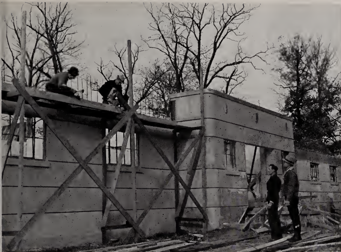
Constructing community youth center.
