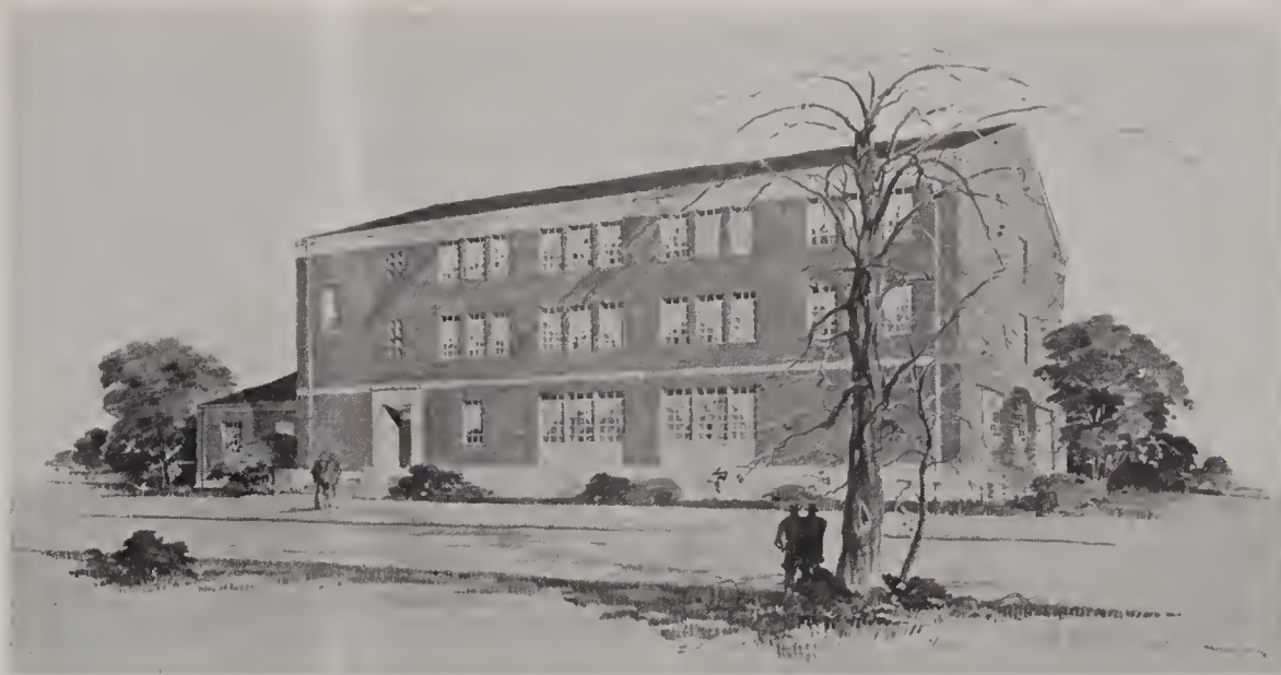
Barracks and school facilities (F. B. I.) Quantico, Va.
