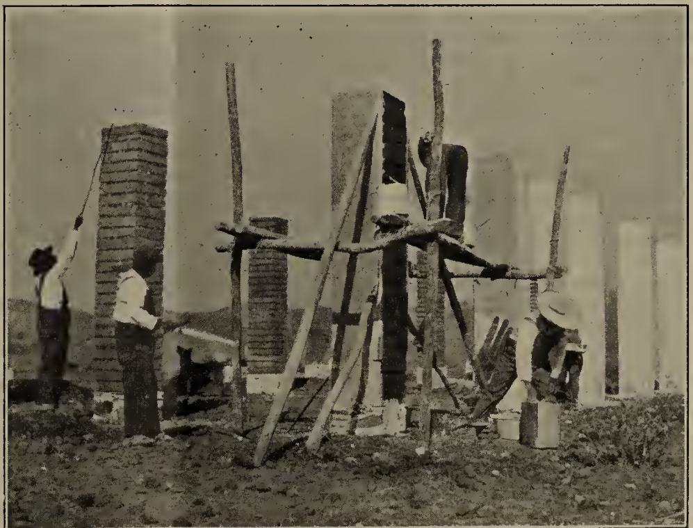
WORK ON THIS SCHOOL WAS STARTED WITHOUT A BOND ISSUE Teachers and pupils sweated in the sun making adobe bricks; they were masons, plasterers, woodsmen, carpenters, blacksmiths, tinsmiths, and even well diggers. It is now an attractive building of one story, stuccoed, painted in white with a red tiled roof.
