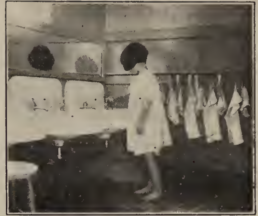
Pantry converted into first-floor toilet room. Bathroom equipped with junior size fixtures; height of basin, 21 inches; of toilet, 10 inches
