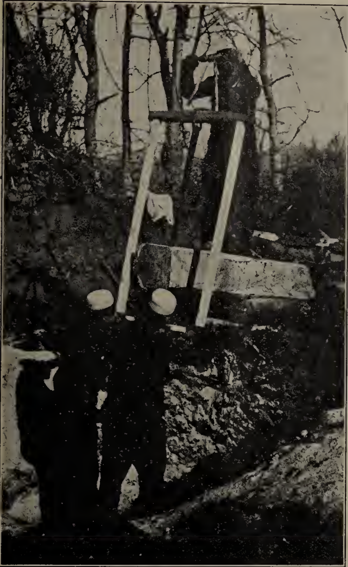
Copyright A. R. C. Boards for the new building were sawed by primitive methods
