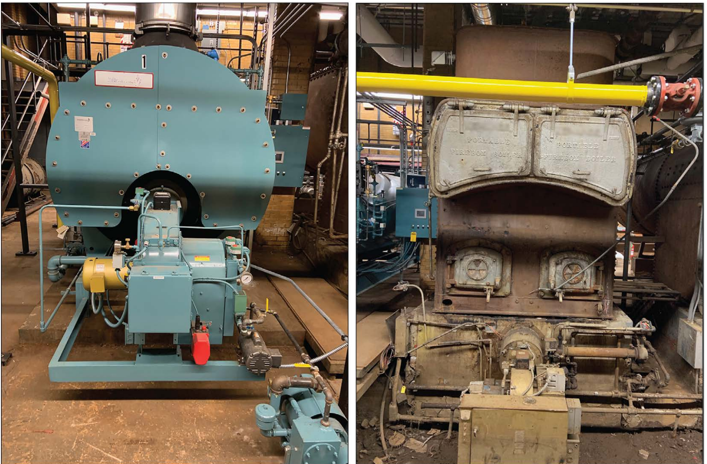
Figure 3: Public School in Rhode Island with One New Boiler (left) and One Original to 1931 Building
