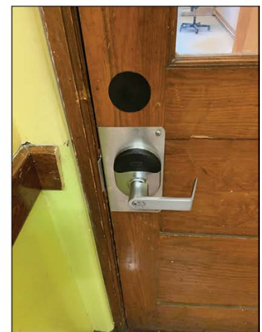
A classroom door with a remote locking mechanism in a Rhode Island school.
