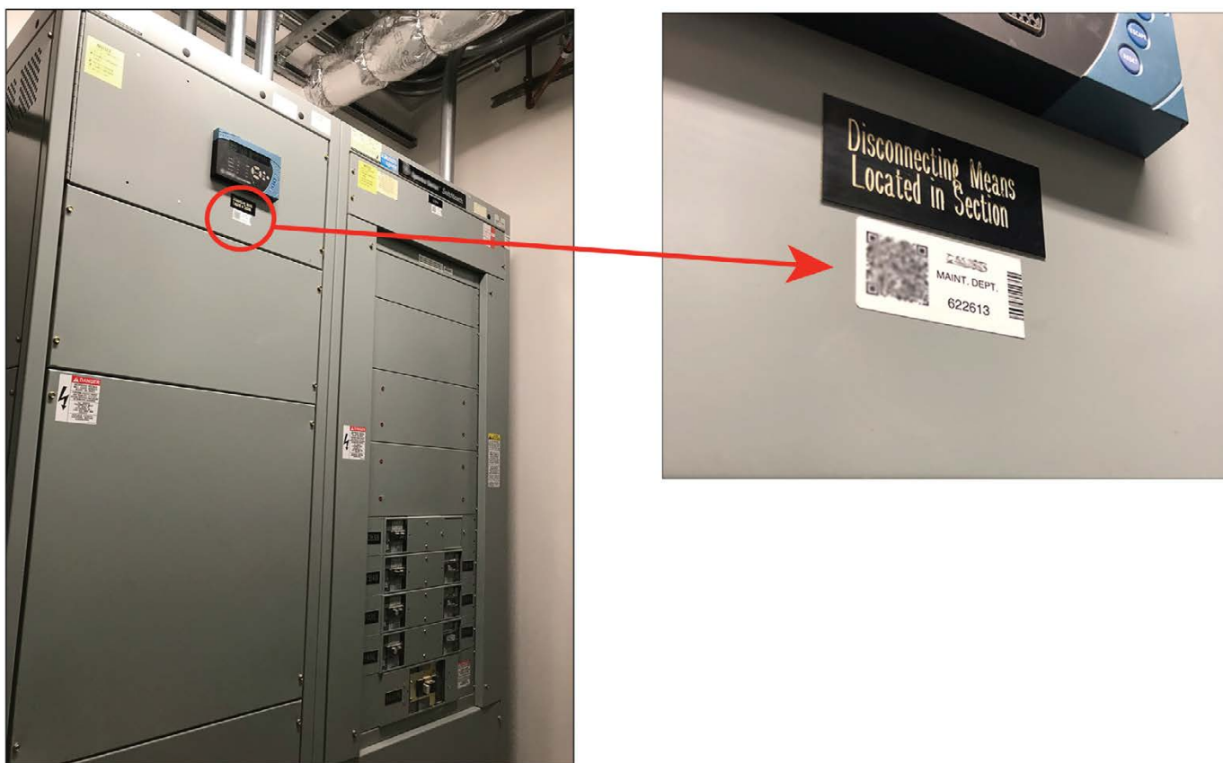
Figure 9: Barcodes Used to Help a California School District Track the Condition of Building Systems in its Public Schools
