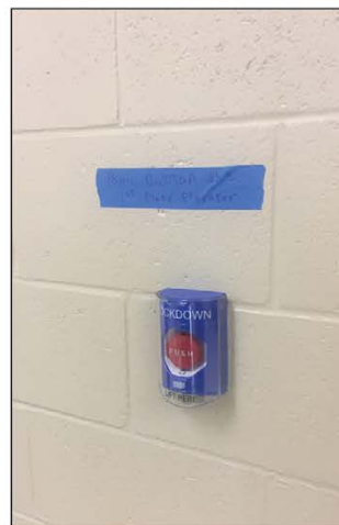
A button that locks exterior doors in the hallway of a Florida school.
